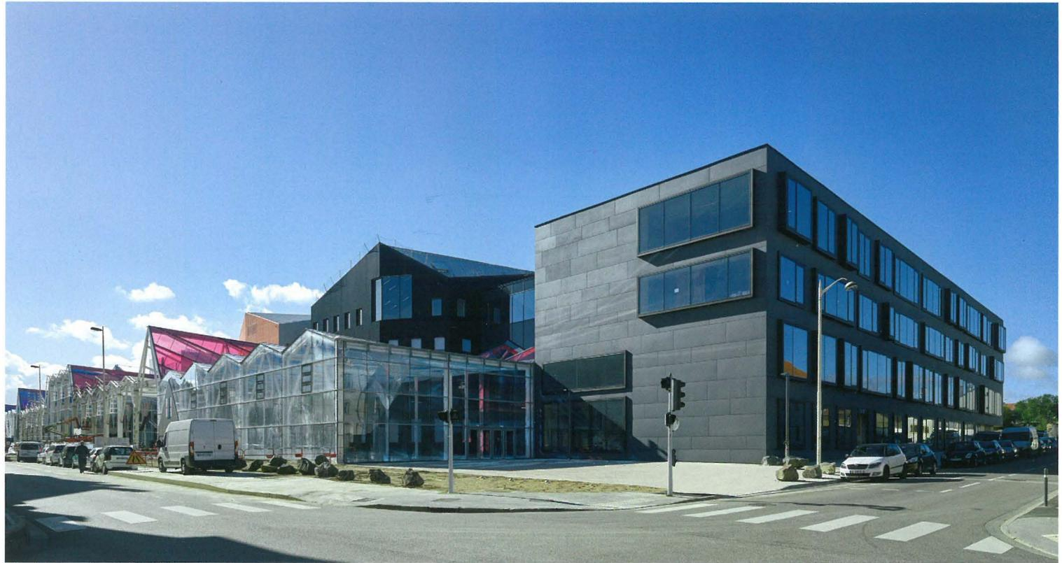
Towards the street junction the simple building volume creates a space-shaping edge. Here the box-like windows that project to different extents from the facade on the long side of the building can exert their full impact. On the short side the dark fibre cement panels dominate. Mounted in a staggered pattern they respond to the storey heights and the box -like windows and are of different heights and lengths.
